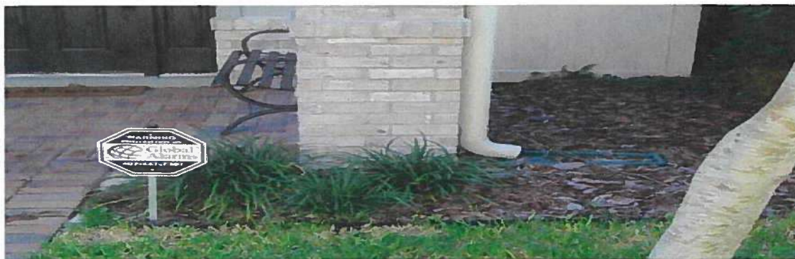
October 18, 2023, Disc PRE1, Photograph 223, JF, 2-unit building, downspout outlets at base of column.
